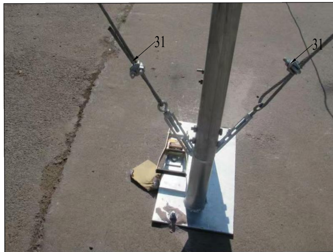
Figure 8 The position of windstabilizers(turnbuckle and cable) at the sidewall.
