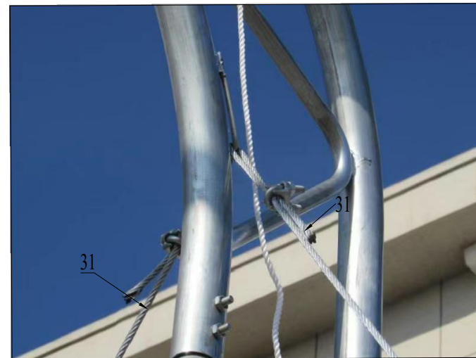
Figure 8 The position of windstabilizers(turnbuckle and cable) at the sidewall.
